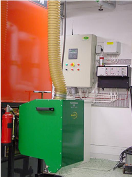
Figure 4.18. The EcoTec 300 kW pellet burner (Sweden)
