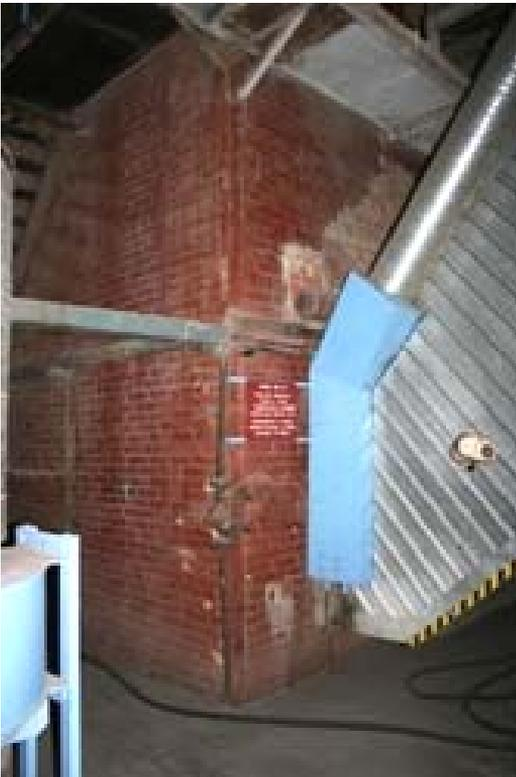
Figure 8.17. Far end of the tertiary air channel, photo by Ü. Kask
