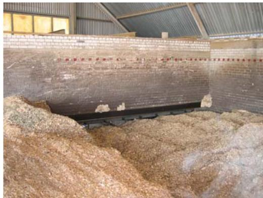
*Figure 8.24. Fuel in the storage section equipped with hydraulic pushers in Võrusoo Boiler Plant, photo by Ü. Kask*
