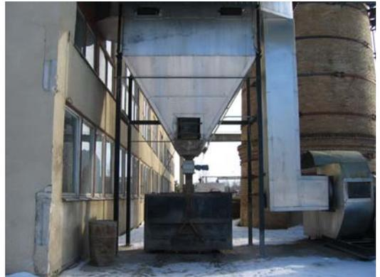
B. Container under the ash hopper. Between the hopper and container an air-lock can be seen.
