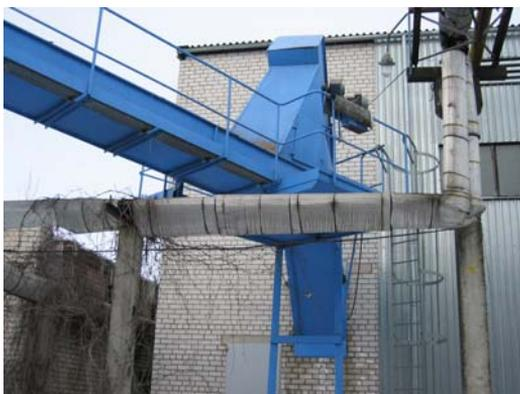
*Figure 8.19. DH pipes obstructed the route planned for the conveyors from the storage to the boiler plant, photo by Ü. Kask*
