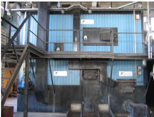
Figure 8.22. Pre-furnace installed in Võrusoo Boiler Plant, photo by Ü. Kask
