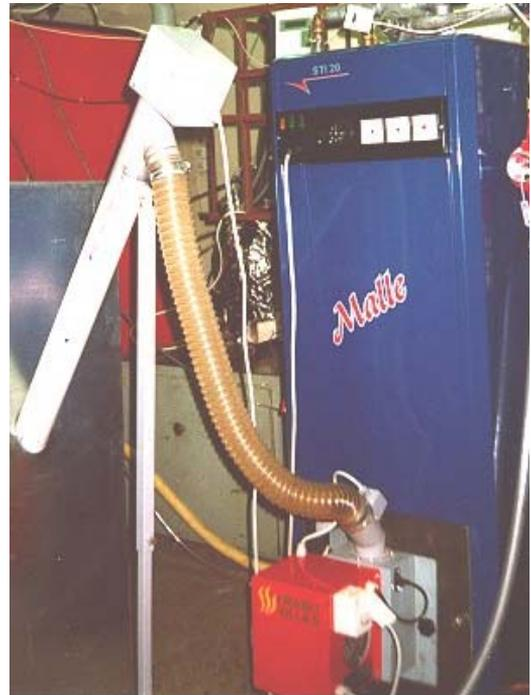
Figure 4.27. The Malle 20 kW boiler (AS Viljandi Metall, Estonia) with the pellet burner Iwabo VillaS and pellet feeding system
