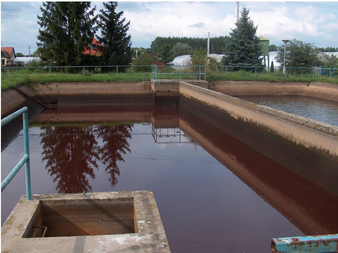
**Figure 1. The collection and drying pools for sludge**
