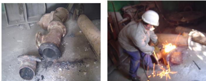
**Figure 2. Cutting of a pipe to remove the Norm material**
