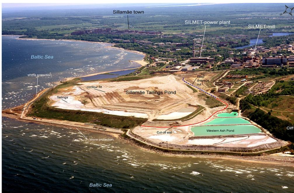
**Figure 6. Sillamäe tailings pond, unremediated in 1999** (source: Wismut and C&E 2001)
