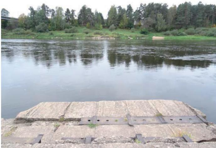
**Figure 36:** At a number of places, it was apparent that the Soviets had expected the interdiction of bridges and had, as a result, placed abutments for pontoon bridges (as was the case at Krāslava near the A6 bridge over the Daugava River) or concrete beds in the river to support movement in the event that bridges were made unusable in the course of conflict.
