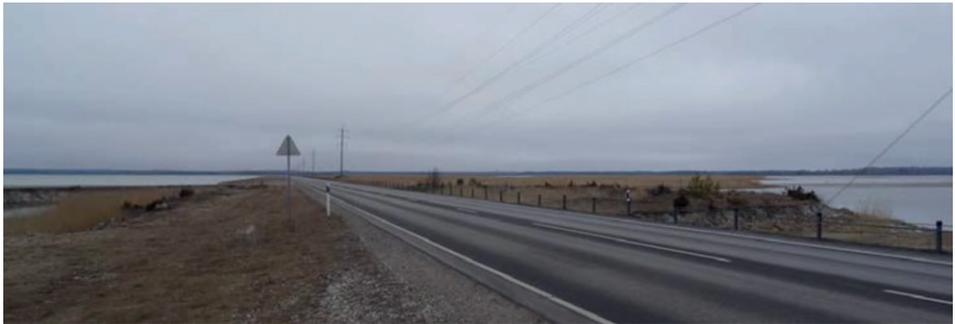
**Figure 71:** While maps tend to depict Saaremaa being connected by Muhu by a bridge, it is actually a causeway that has been constructed through marshland between the two islands. Therefore, this land transportation link would be far more difficult to cut than it would be to take down a bridge. Another implication is that it is impossible to travel via water directly from the Gulf of Rīga and the Väinameri.
