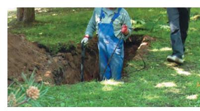
Communications cables damaged during the excavation works
