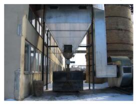
**B.** Container under the ash hopper. Between the hopper and container an airlock can be seen.
