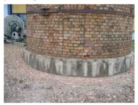
Figure 8.12. Brick crumbs at the foot of crumbling stack, photo by Ü. Kask
