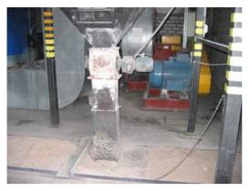
Figure 8.36. Multicyclone foundation and concrete channel cover, photo by Ü. Kask
