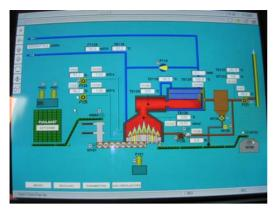
Figure 8.43. Scheme of Peetri Boiler Plant with the operation parameters displayed on the server screen, photo by Ü. Kask
