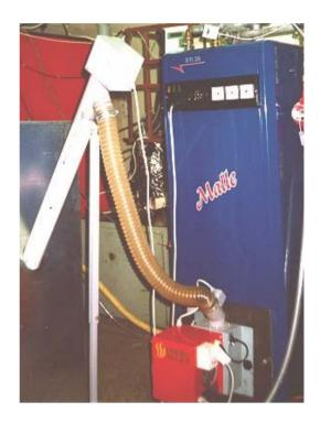
Figure 4.27. The Malle 20 kW boiler (AS Viljandi Metall, Estonia) with the pellet burner Iwabo VillaS and pellet feeding system
