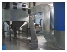
Figure 8.41. Multicyclone and ash conveyor, photo by Ü. Kask
