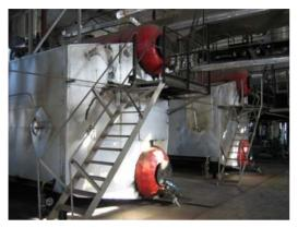
Figure 8.21. The DE-type boilers in Võrusoo Boiler Plant, rear view, photo by Ü. Kask
