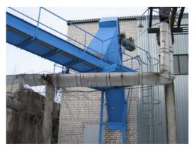
Figure 8.19. DH pipes obstructed the route planned for the conveyors from the storage to the boiler plant, photo by Ü. Kask
