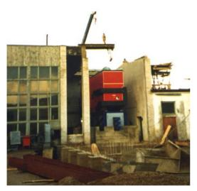
Figure 8.6. Assembly of the complex biofuel boiler unit in Tehnika Boiler Plant in Türi, photo by V. Vares
