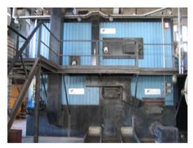
Figure 8.22. Pre-furnace installed in Võrusoo Boiler Plant, photo by Ü. Kask
