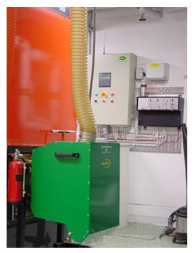
Figure 4.18. The EcoTec 300 kW pellet burner (Sweden)
