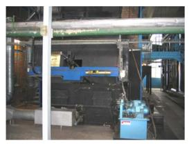
Figure 8.26. Front view of the reconstructed DKVR-type boiler, photo by Ü. Kask
