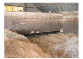
Figure 8.24. Fuel in the storage section equipped with hydraulic pushers in Võrusoo Boiler Plant, photo by Ü. Kask
