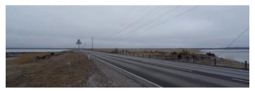
**Figure 71:** While maps tend to depict Saaremaa being connected by Muhu by a bridge, it is actually a causeway that has been constructed through marshland between the two islands. Therefore, this land transportation link would be far more difficult to cut than it would be to take down a bridge. Another implication is that it is impossible to travel via water directly from the Gulf of Rīga and the Väinameri.
