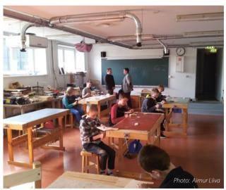
The powerful wood dust collection system in the handicraft and technology class at Kiili Upper Secondary School prevents the wood dust from causing damage to health.
