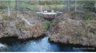
The new cofferdam in Viru Bog prevents water outflow from the natural bog; the restored area is separated from the natural bog by a ditch.
