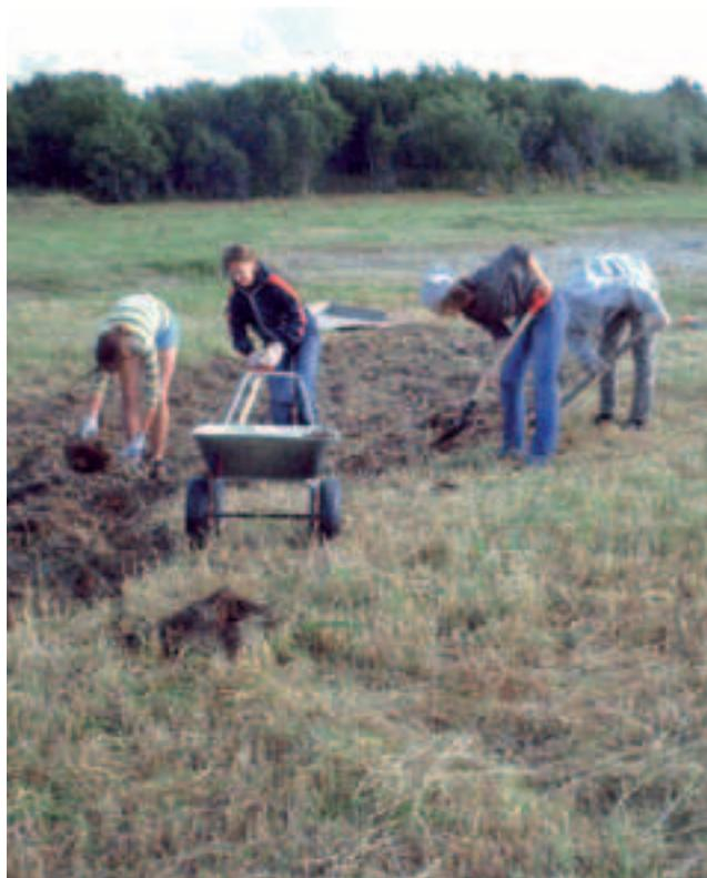
**Best result was achieved with cutting the reed and removing it first and digging the mud and roots of reed out afterwards.**
