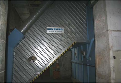
Figure 8.16. Fire pass between the pre-furnace and boiler, photo by Ü. Kask
