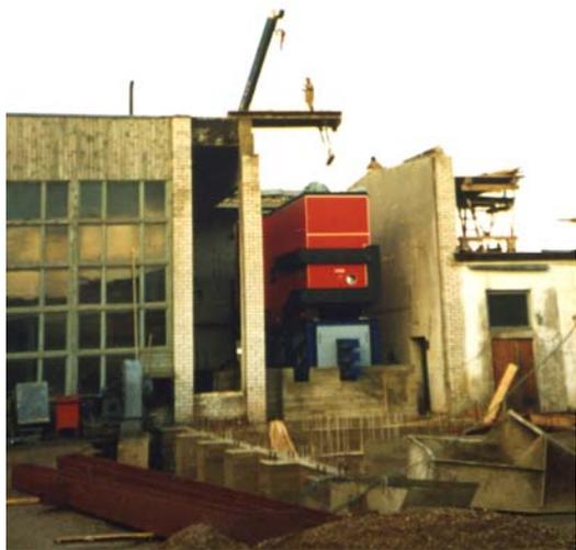
*Figure 8.6. Assembly of the complex biofuel boiler unit in Tehnika Boiler Plant in Tūri, photo by V. Vares*
